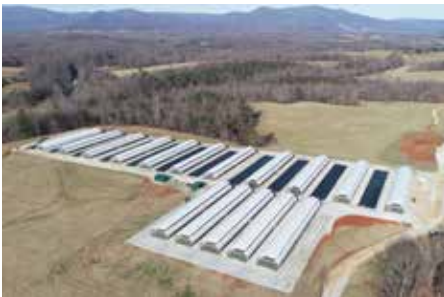
2023 Greenhouse expansion at our Randolph Farm location
